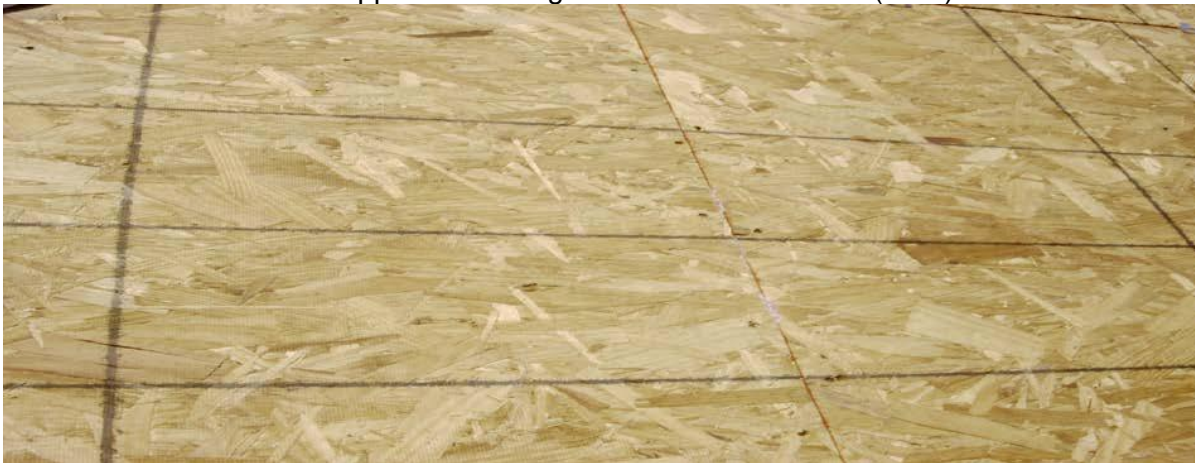
New Deck Application Using Oriented Strand Board (OSB)
