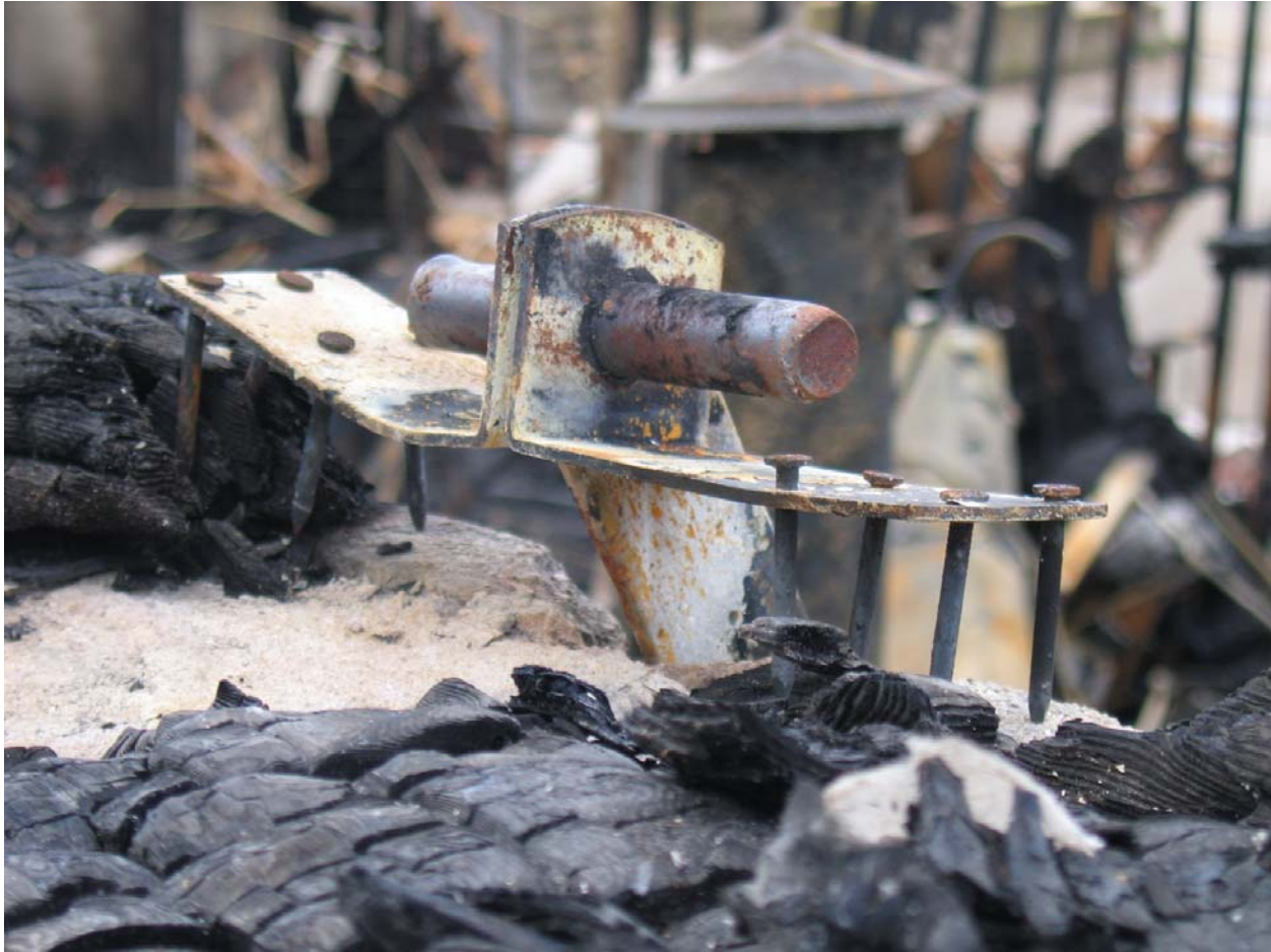
Figure 3. Roof truss attachment to east wall (Photo by SFMO)
