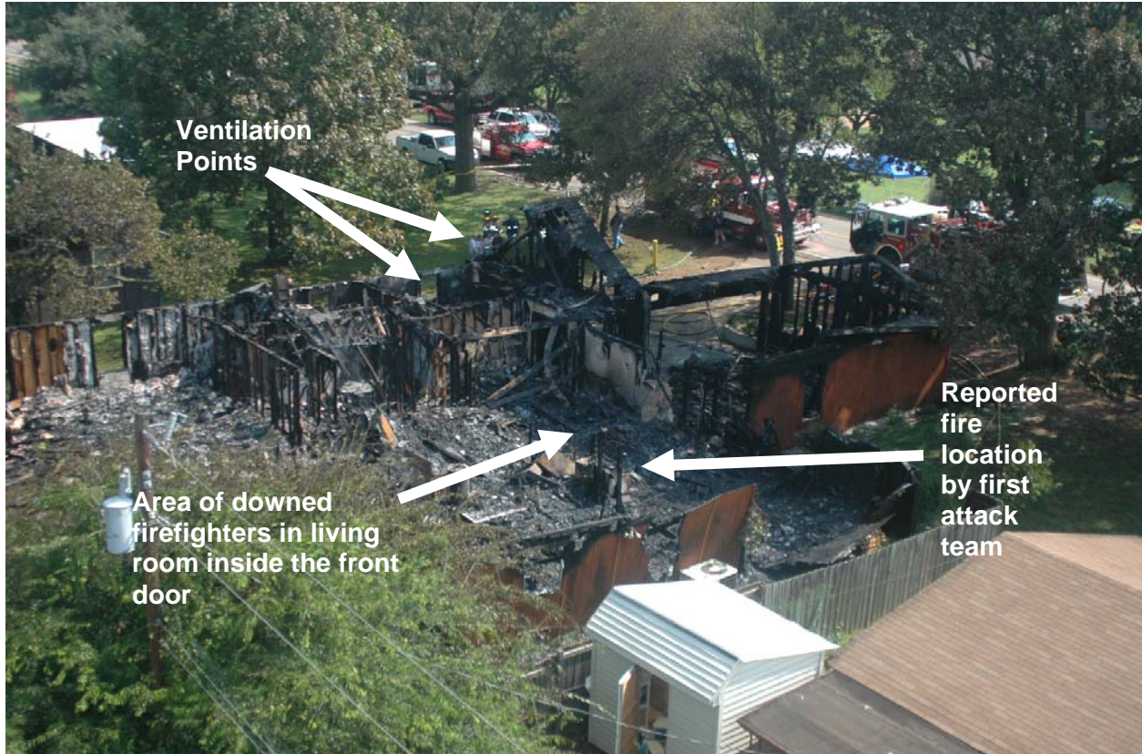
View of the scene from the southwest (Photo by Smith County Fire Marshal)
