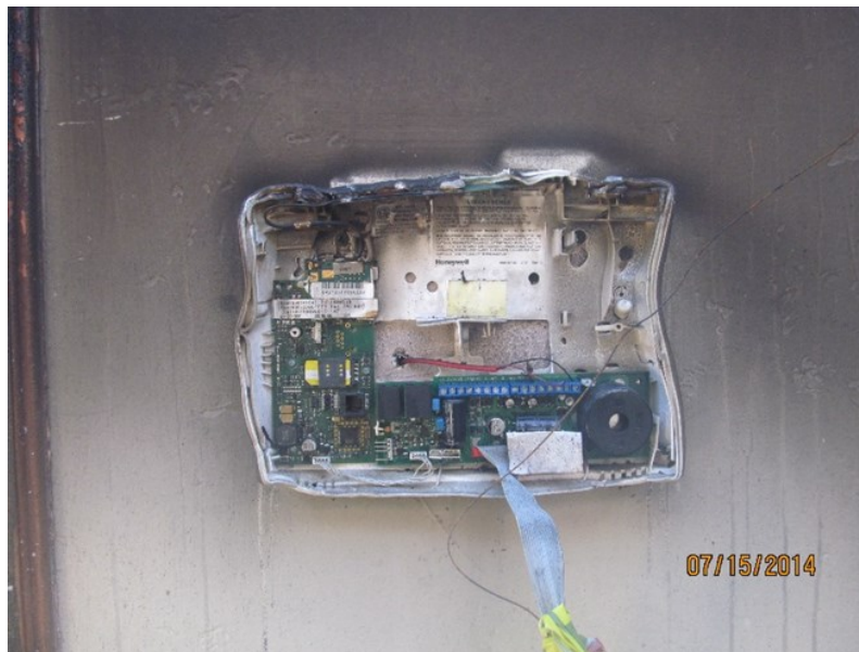
The remains of the alarm system attached to an interior wall.
