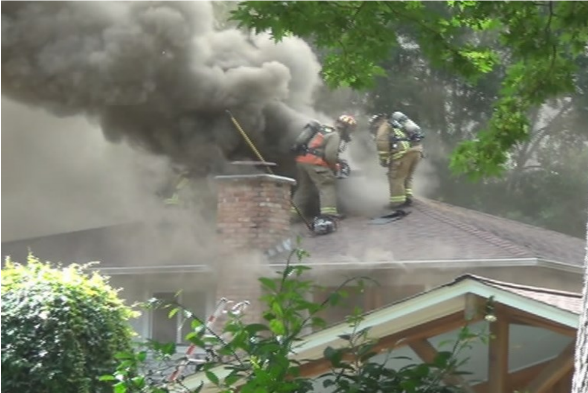
Ladder 102 is on the roof for ventilation. Screenshot of video provided by Houston FD. The double doors below them open into the room where Firefighter Groover was located.
