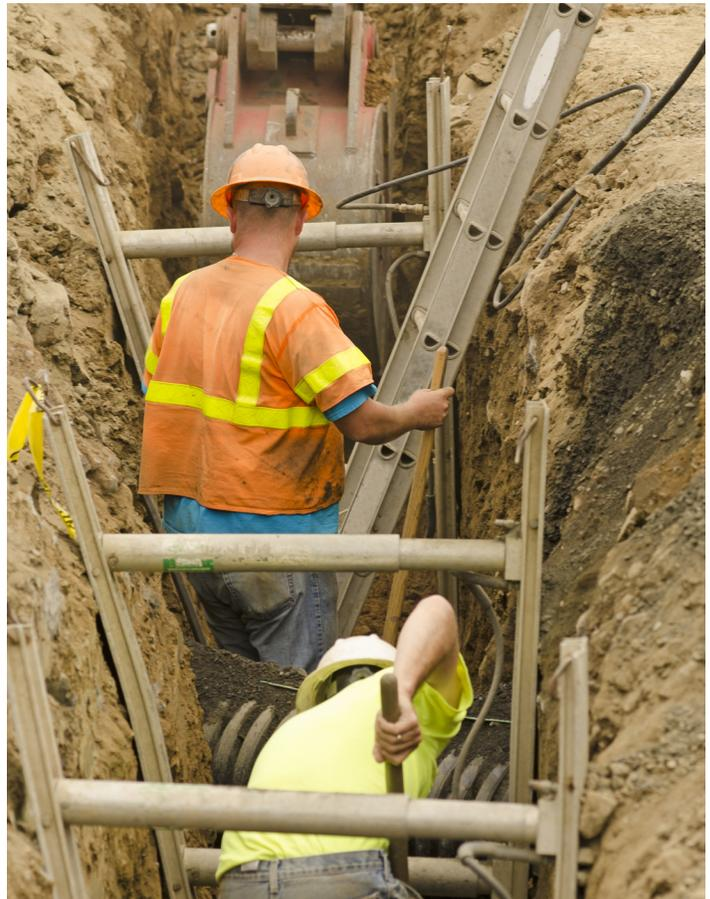
movement if the earth starts to shift. These steps protect workers from the pressure and weight of soil in the event of a cave-in. One cubic yard of soil can weigh as much as a car: 3,000 pounds.<sup>1</sup>
