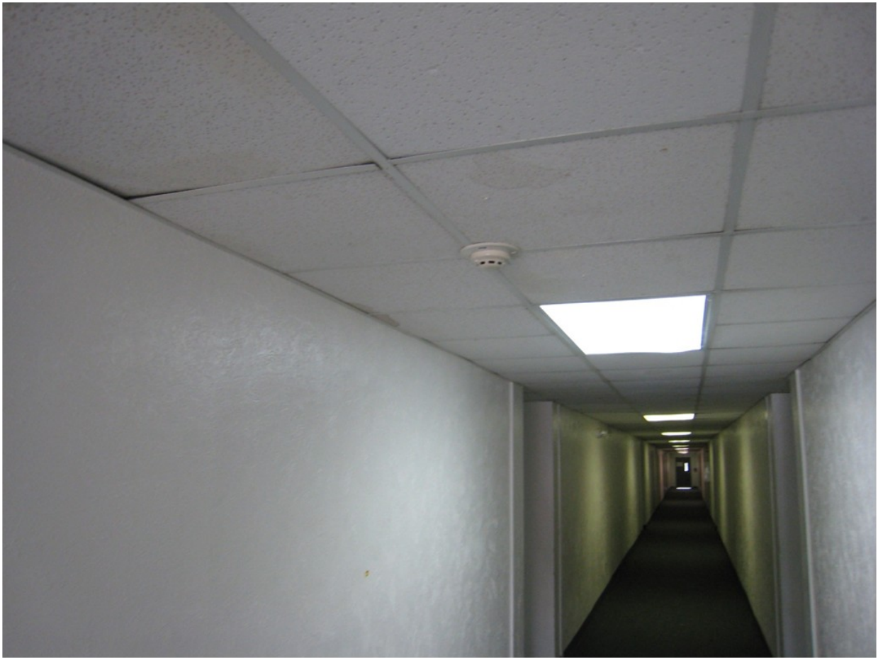
View of corridor in exemplar structure
