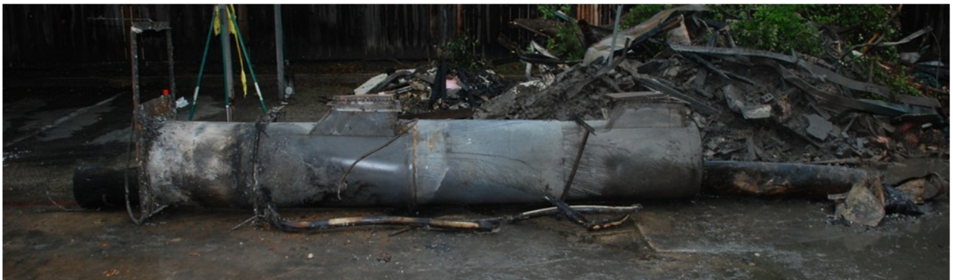
Trash chute with first floor at left and attic vent at right
