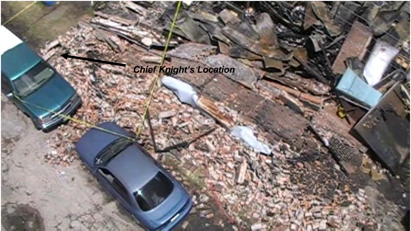
Photograph of the south end collapse zone
