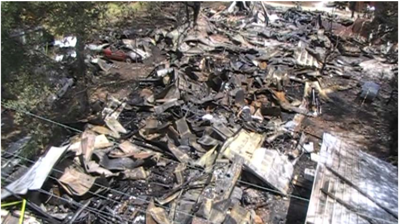
Overhead photograph from the south end of the site.
