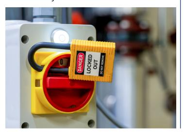
energy entering the system. In most cases, there will still be residual energy left in the lines as pressurized fluid. This residual energy can be removed by bleeding the lines through pressure relief valves. Contact the manufacturer for more specific details.
